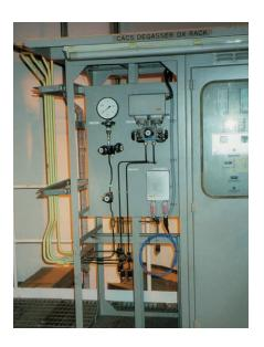
At the station, there are several recirculating loops gas circulator auxiliary coolingsystem, reactor bypass gas plant, diagrid support skirt and pressure vessel cooling, etc. The degassers remove hydrogen and oxygen released as the cooling water undergoes radiolysis.
