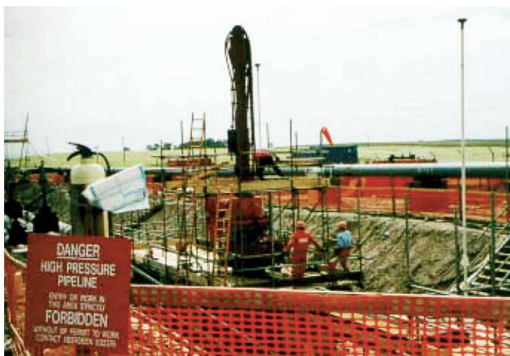
Installation of one of the new pumping stations in progress on the B.P. Forties Pipeline, without interrupting the flow of crude!
