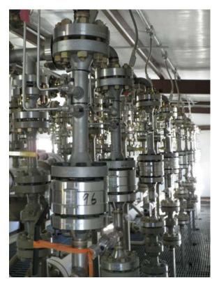
Figure 2: Installed V-Cone Flowmeters
