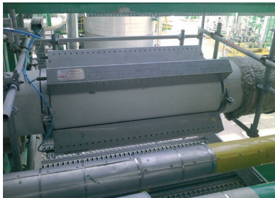
Kashagan Field – SlugMaster Time of Flight Transducers
