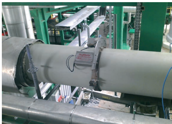
Kashagan Field – SlugMaster Reflexor Transducers
